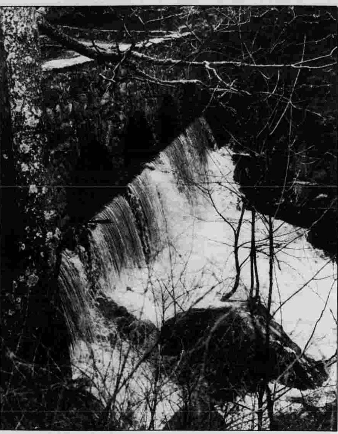
HIGH WATER — The warm January weather and recent rains have combined to raise local rivers and streams. The overflow spills over the dam at Highland Park Falls Friday afternoon.
